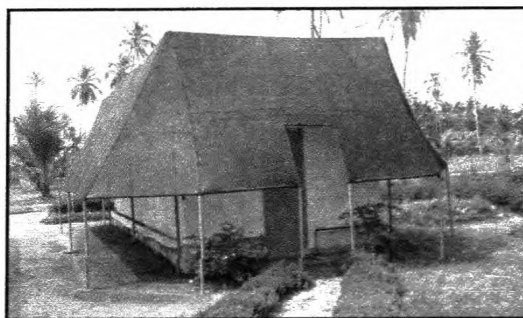
Figure 2. Growing house with new cladding material
