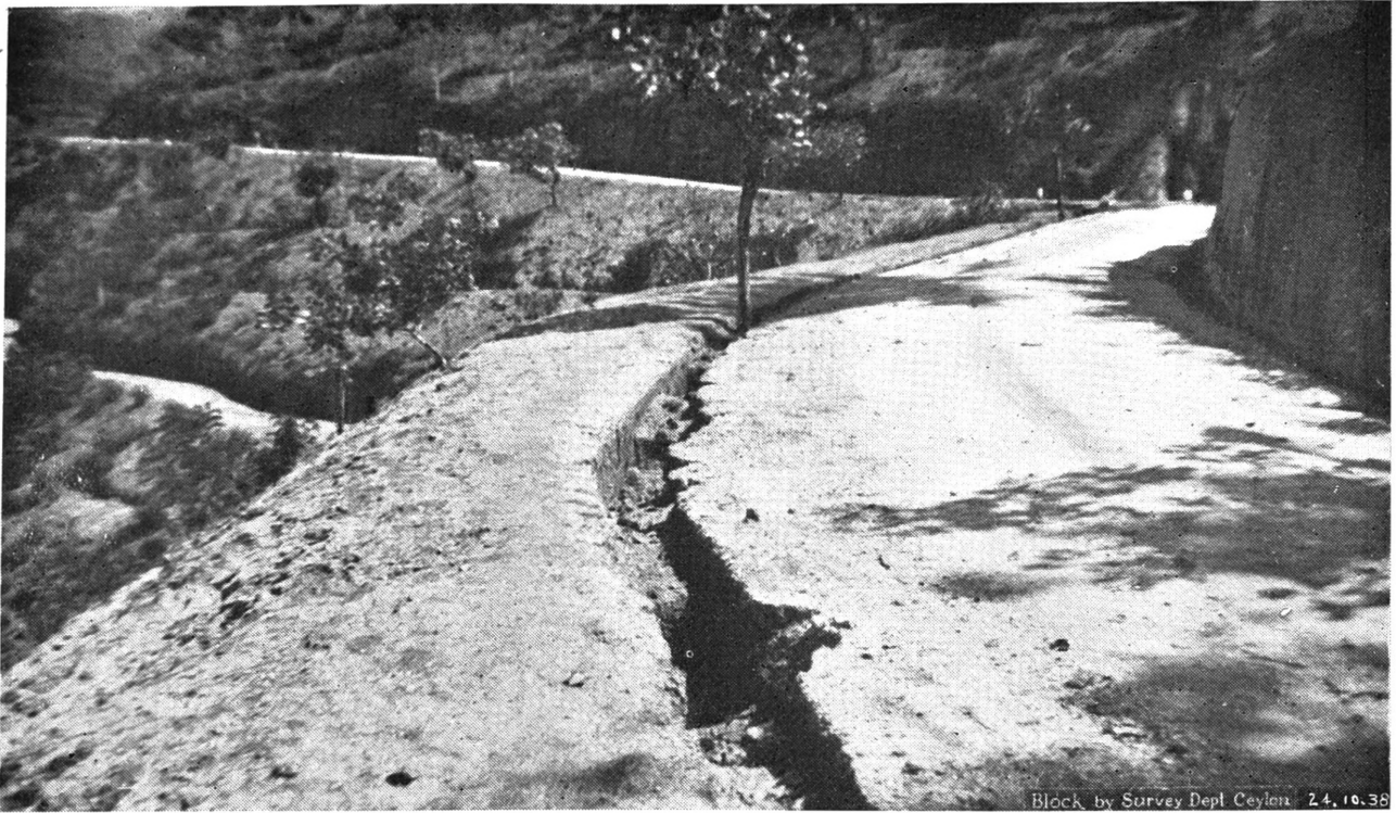
FIG. V.—DRAIN-SIDE EROSION.
