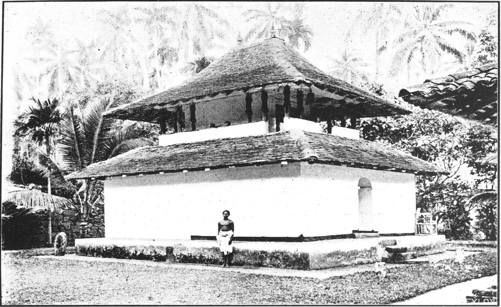
No. 5.—DIYASUNNATA VIHARE, RAMBUKKANA, VIEW FROM THE EAST.
