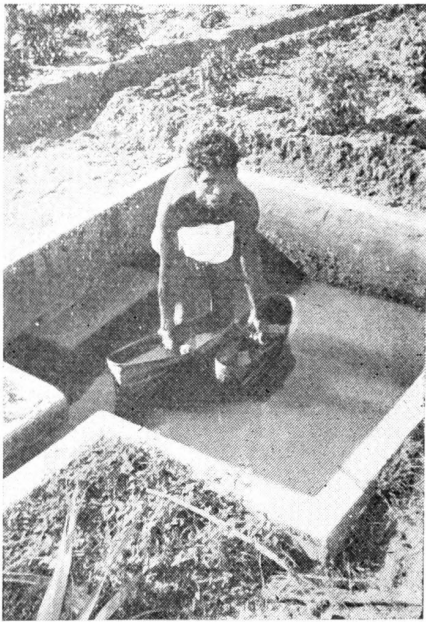
PHOTO 3.—Lined pond for irrigation.
