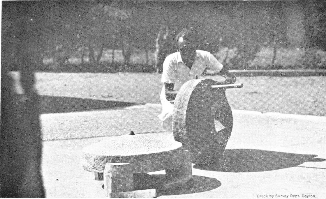
FIG. 9.—SIDE VIEW OF THE COMMERCIAL MODEL OF DHAL-SPLITTING MILL.
